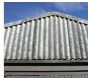
Asbestos cement panels
